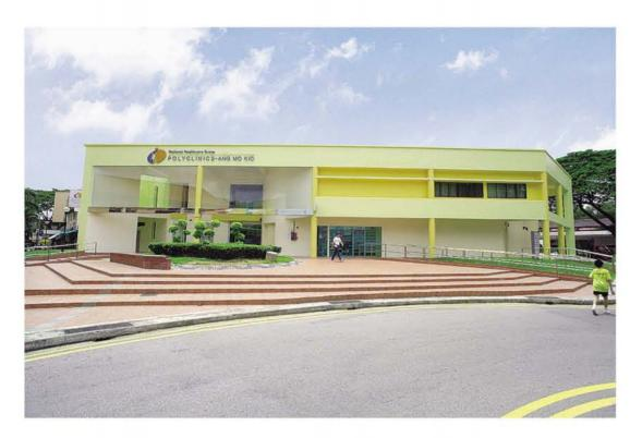
Total floor area is 3,400 m² and 2 stories. Construction was completed in 2003. The VRV system was selected for this clinic because its signature energy-saving characteristics were appropriate to customer needs. Also, VRV permits piping lengths of up to 100 m between the indoor and outdoor units, offering a degree of design freedom that was appreciated by the customer. The clinic was also impressed with the low cost of maintenance a VRV system requires.
