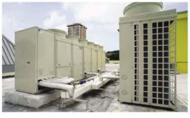
Air-conditioning capacity is 710 Hp, or 2064 kW, 587 USRT.
