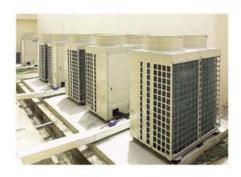
Air-conditioning capacity is 290 Hp, or 843 kW, 240 USRT.
